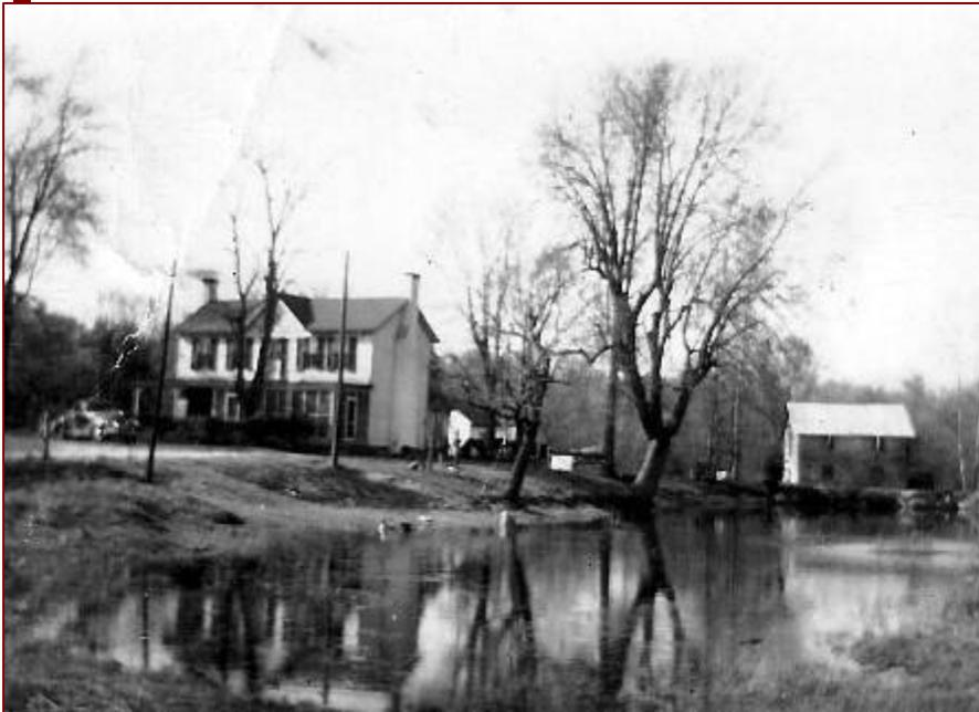
**The mill is a two storied wooden structure, rectangular in shape, with a gable roof. There is a good metal roof on the mill that protects the mill from the weather. The first level framing of the mill indicates that the mill was built during the first quarter of the 19th Century. The mill was extensively remodeled in 1923. The Fitz steel water wheel was added as well as the 2nd level of the mill. A new roof, new siding and repairs to the foundation were made.**
